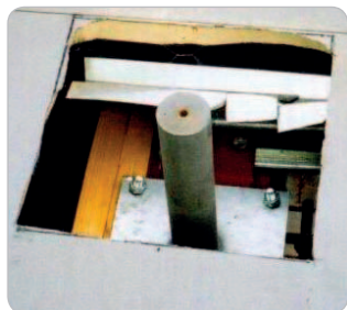
Traditional 'through the roof' post
